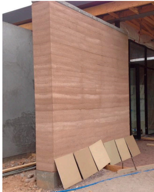
Figure 1. Wall made from compacted earth. The compacted layers of mixed soil are shown.
