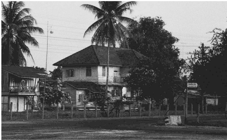
The building that once housed the Imperial Japanese Consulate in Songkhla (photo by the author March 1968)
