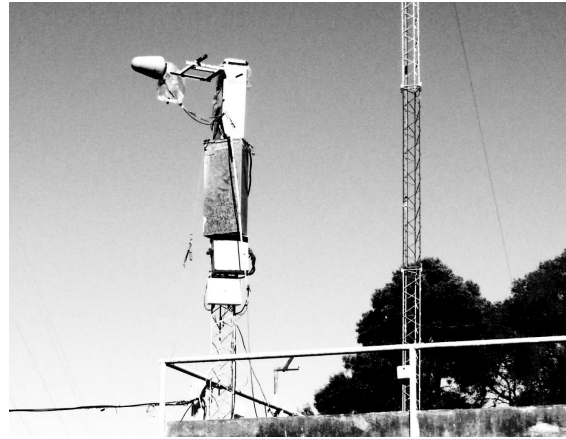
Fig. 2 Foto of pedestal mounted on the roof of the operation house with the broadband antenna from the Wettzell RFI monitoring system. This configuration was used almost continuously from September 14 until October 14, 2012.
