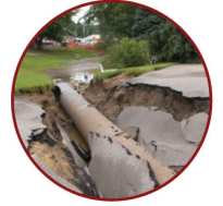
FLOODING/EROSION ROAD COLLAPSE
