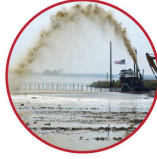
THIN LAYER PLACEMENT
