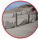
BROKEN SAND FENCES
