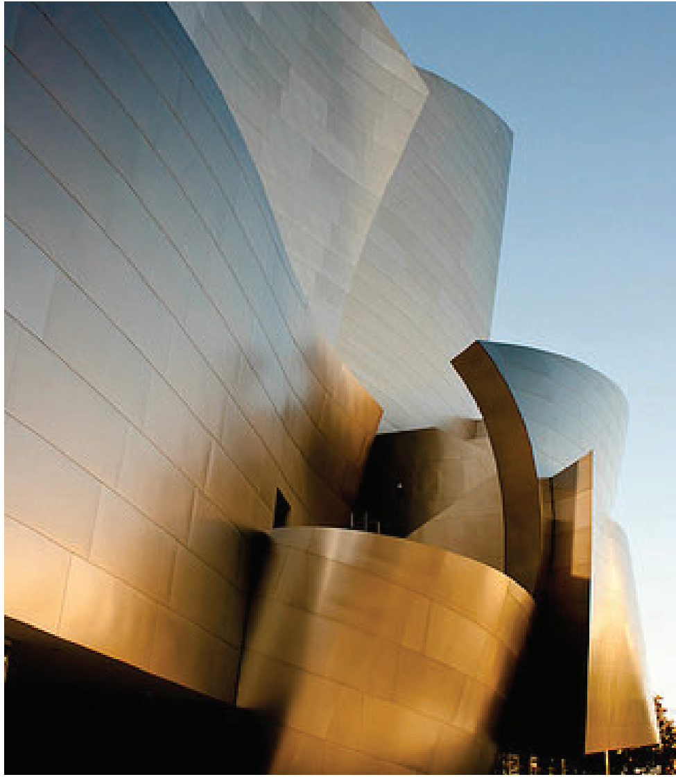
Fig. 42 - View of Curving panels
