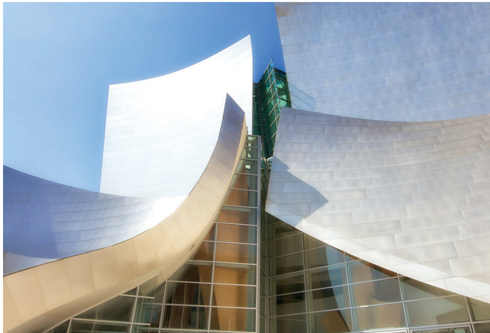
Fig. 46 - View of Entrance
