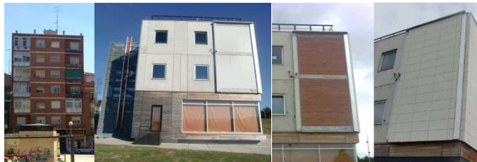
Figure 3: Left: Building with brick façade, Center-left: Calibration façade test configuration in KUBIK (phase 0), Center-right: Brick façade test configuration in KUBIK (phase 1), Right: Ventiladed façade solution in KUBIK (phase 2)
