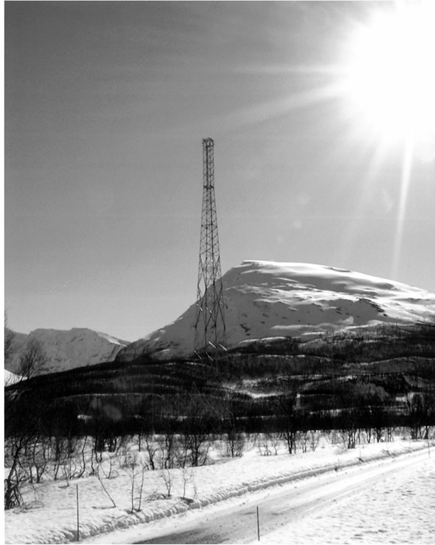
Fig. 8. The current transmitter antenna arrangement at Ramfjordmoen (Photo: Chris Hall).
