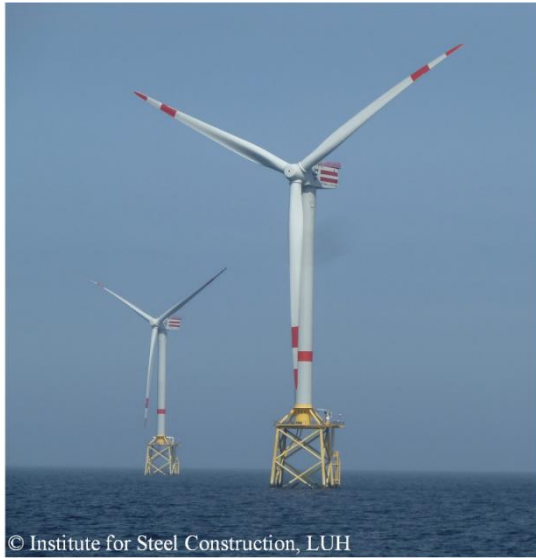
Figure 1. Offshore wind energy turbine with jacket support structure from the offshore wind farm alpha ventus
