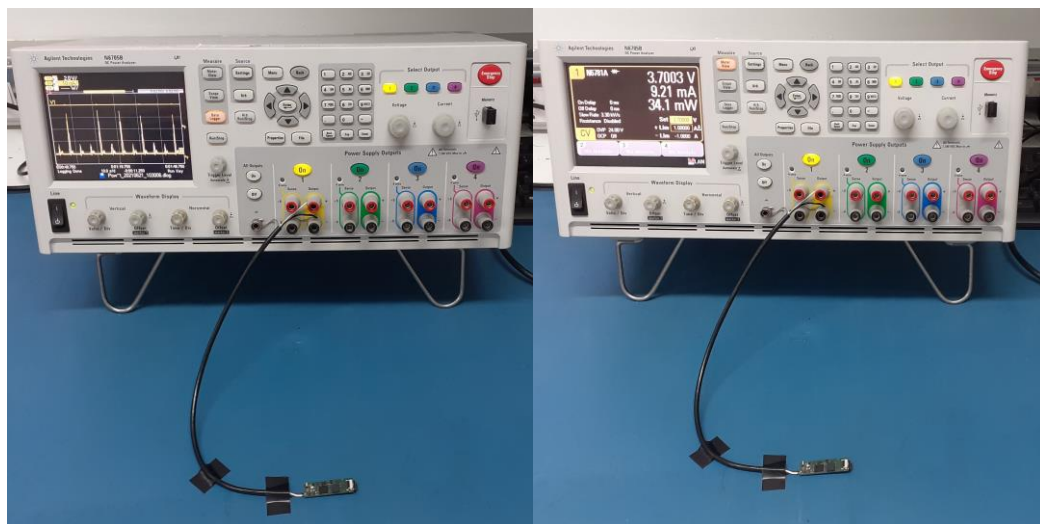
Figure 40 - Power consumption measurement of battery lifetime using a DC Power Analyser.
