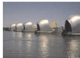
Figure 14: The Thames Barrier.
