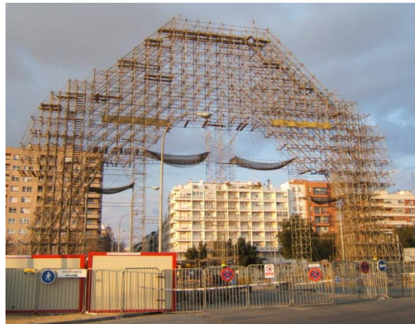
Figure 2. Spatial structure during the building process.
