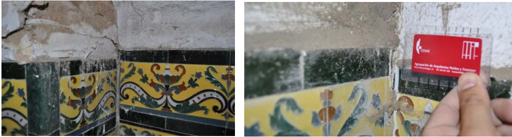
Figures 2 y 3. Offset between tiled baseboards.
