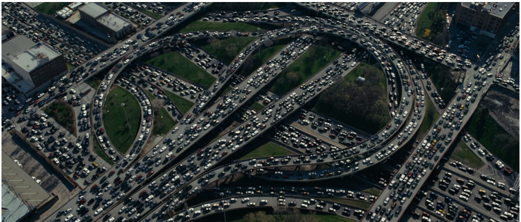
Figure 1.1: Traffic congestion during the 2010 China National Highway 110 Traffic Jam.
