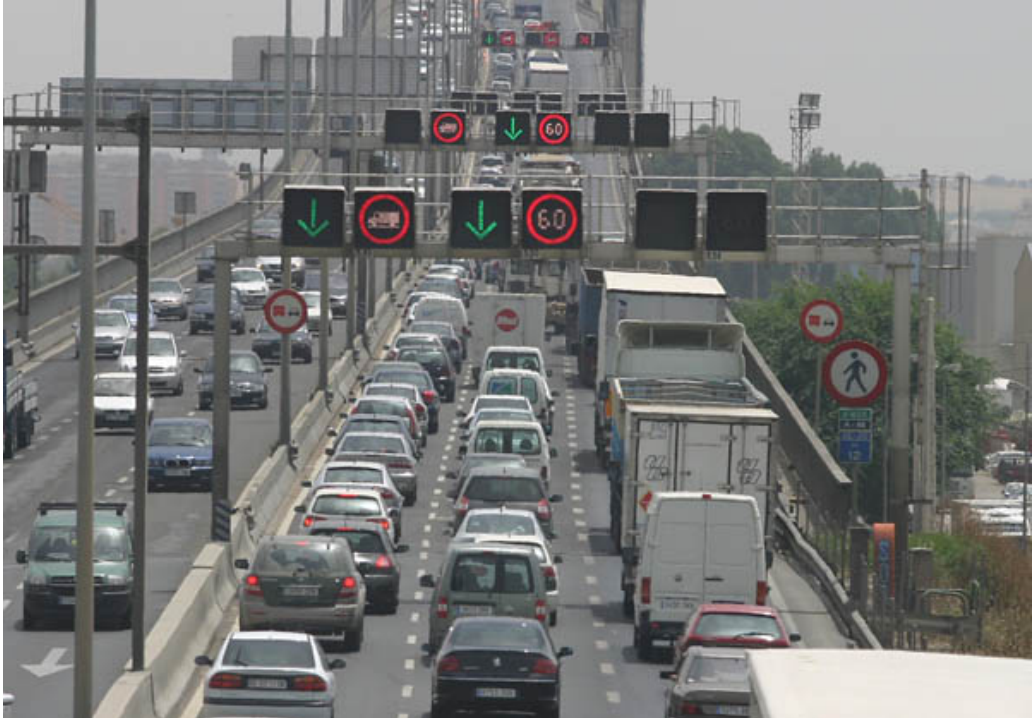
Figure 2.7: Traffic jam on Centenario Bridge, Seville, Spain
