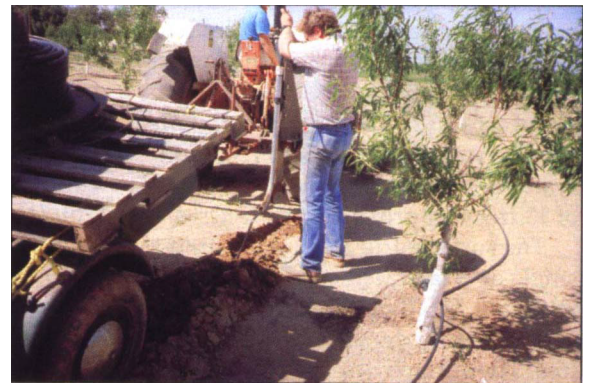
Two configurations of subsurface drip were installed 16 inches deep: a single lateral line, 2 feet from the tree row, and two lateral lines per tree row, each 4 feet from the trees.
