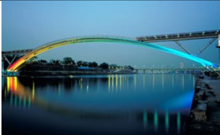
Fig. 2.25. Views of the completed footbridge of peace in South Korea [Brouwer, 2001]
