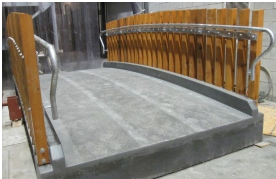
Fig. 4: As final preparation before shipping to the jobsite, wooden and steel railings were attached to the UHPGC curbs
