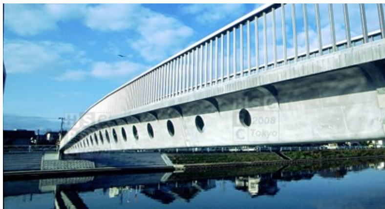
Fig. 2.26. Views of the completed Sakata Mirai footbridge in Japan [Tanaka et al., 2002]
