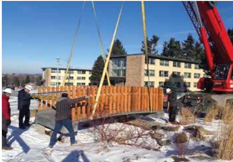
Figure 2. UHPGC Footbridge built at the University of Sherbrooke
