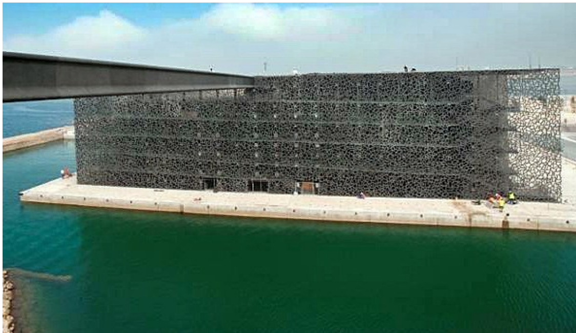
Fig. 2.29: MUSEUM, Marseille, France with UHPC lattice facade, roof and footbridge.
