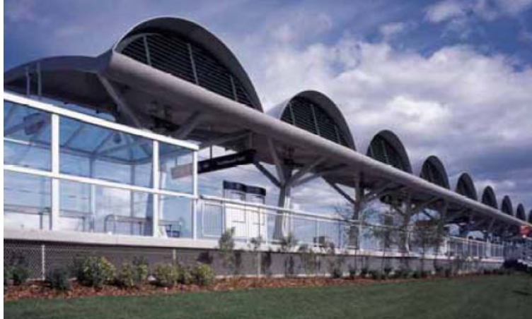
Fig. 2.27. Shawnessy LRT station with UHPC canopies [Perry, 2006]
