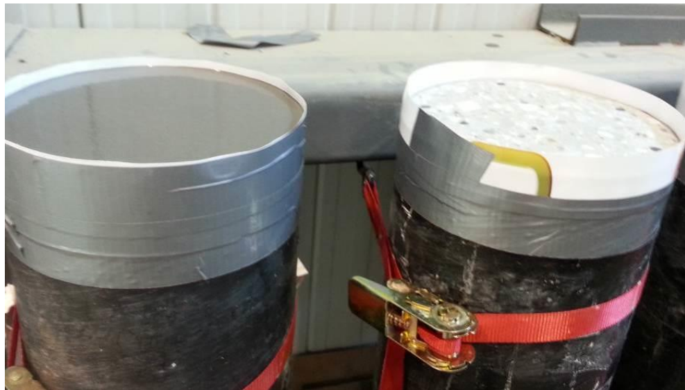
Figure 3.13: Column capping preparation
