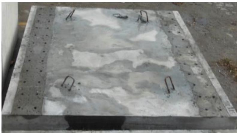
Figure 3–23: Concrete deck slabs after de-molding
