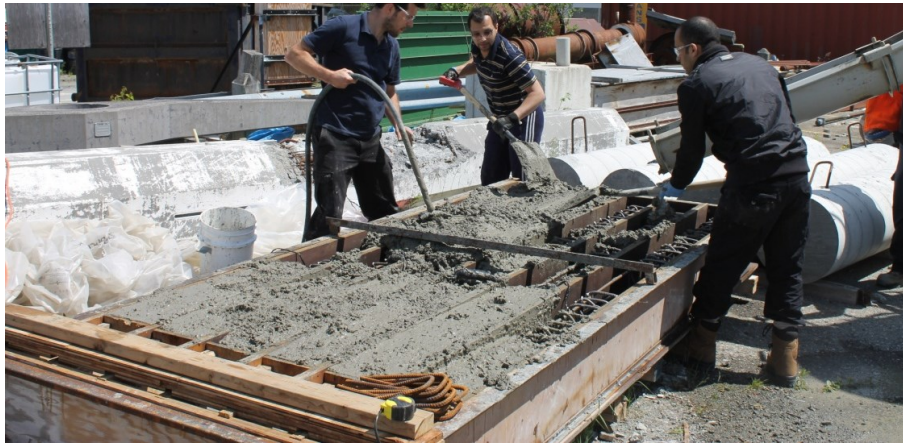
Figure 3–36: Beams during concrete casting
