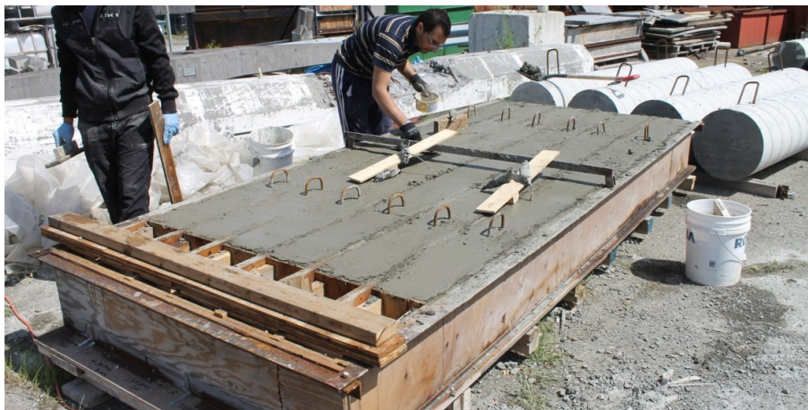
Figure 3–37: Leveling of concrete surface
