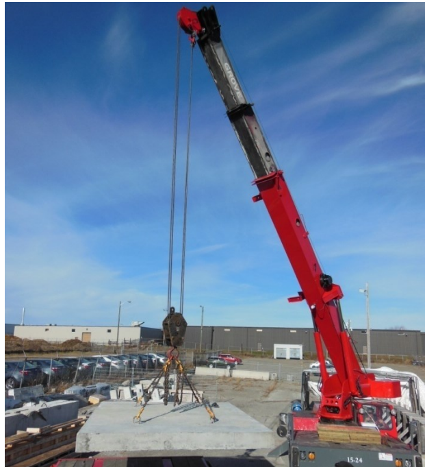
Figure 3–22: De-molding of the concrete deck slabs
