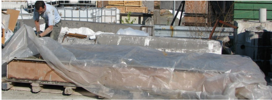
Figure 3–38: Curing of the concrete beams
