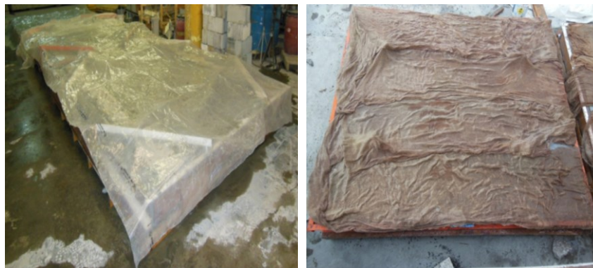
Figure 3–21: Curing of the concrete deck slabs
