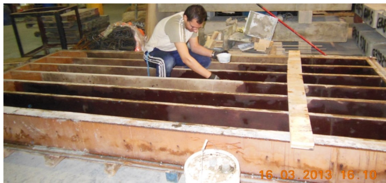
Figure 3–33: Painting of the wooden formwork with oil
