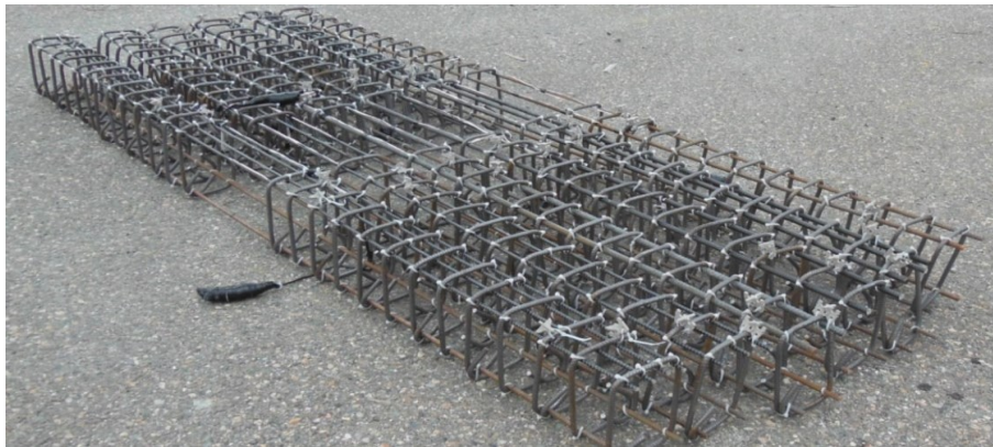
Figure 3–34: Assembled cages
