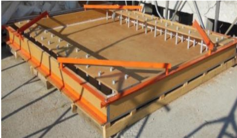
Figure 3–16: The wooden formwork
