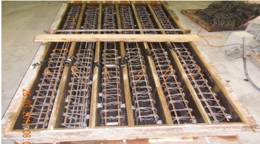
Figure 3–35: Cages of the beams inside the formwork (Before concrete casting)
