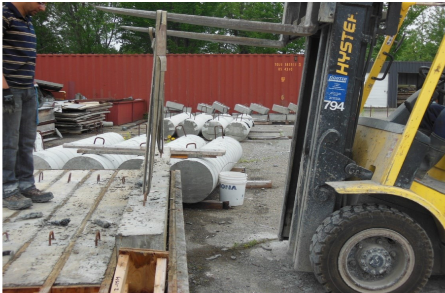
Figure 3–39: De-molding of concrete beams
