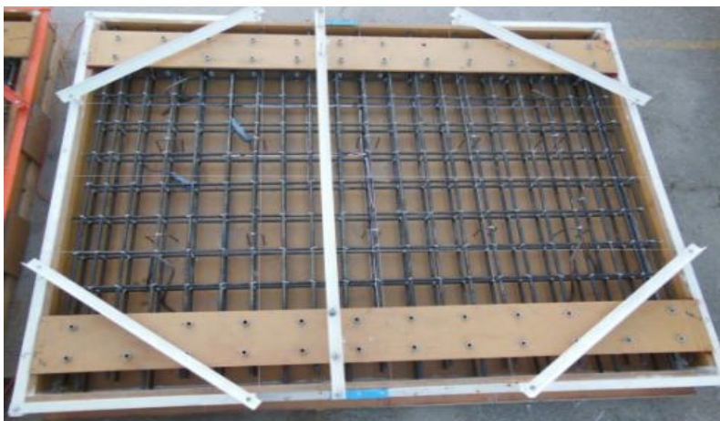
Figure 3–18: Cages inside the formwork (before concrete casting)
