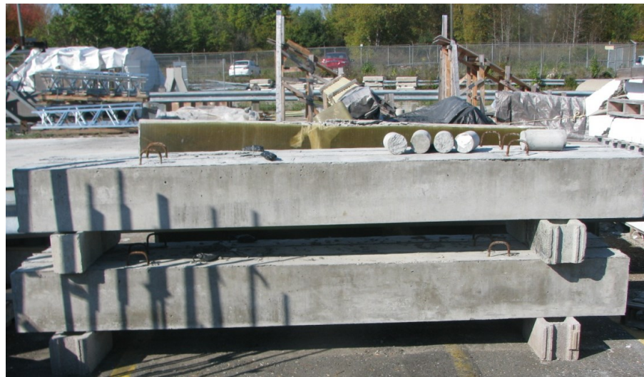
Figure 3–40: Concrete beams after de-molding
