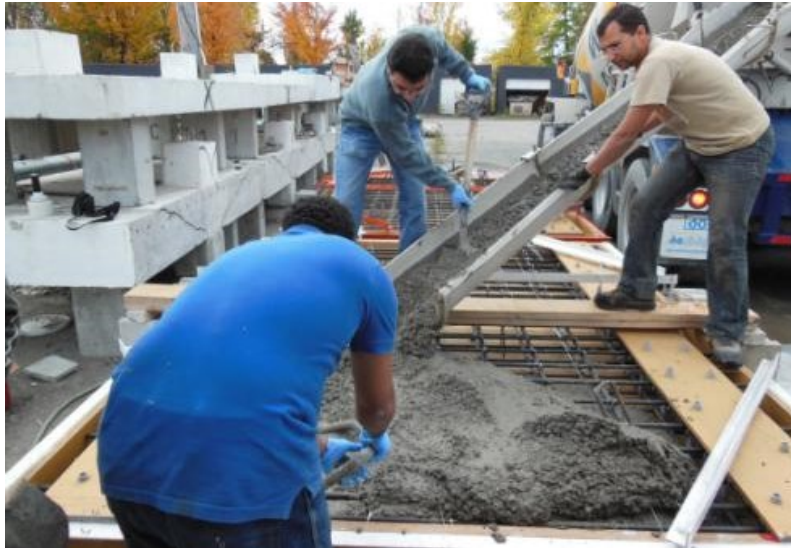
Figure 3–19: Deck slabs during concrete casting
