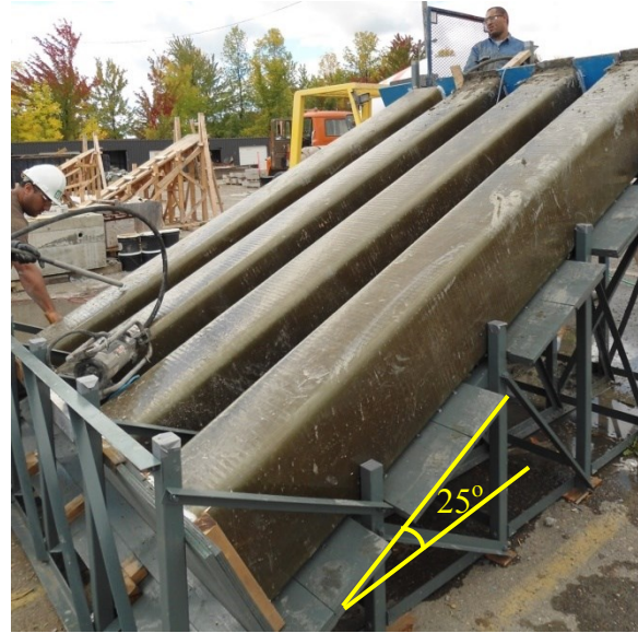
(b) Inclined frames for CFFT beams
