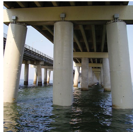
(b) CFFTs in Marine structures
