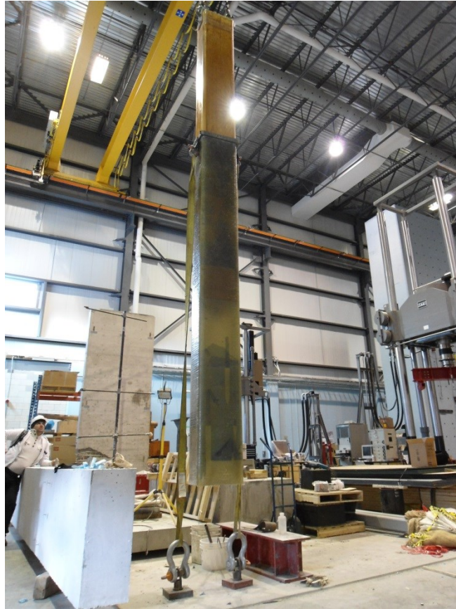
Figure 3.5 – Removing the mandrel
