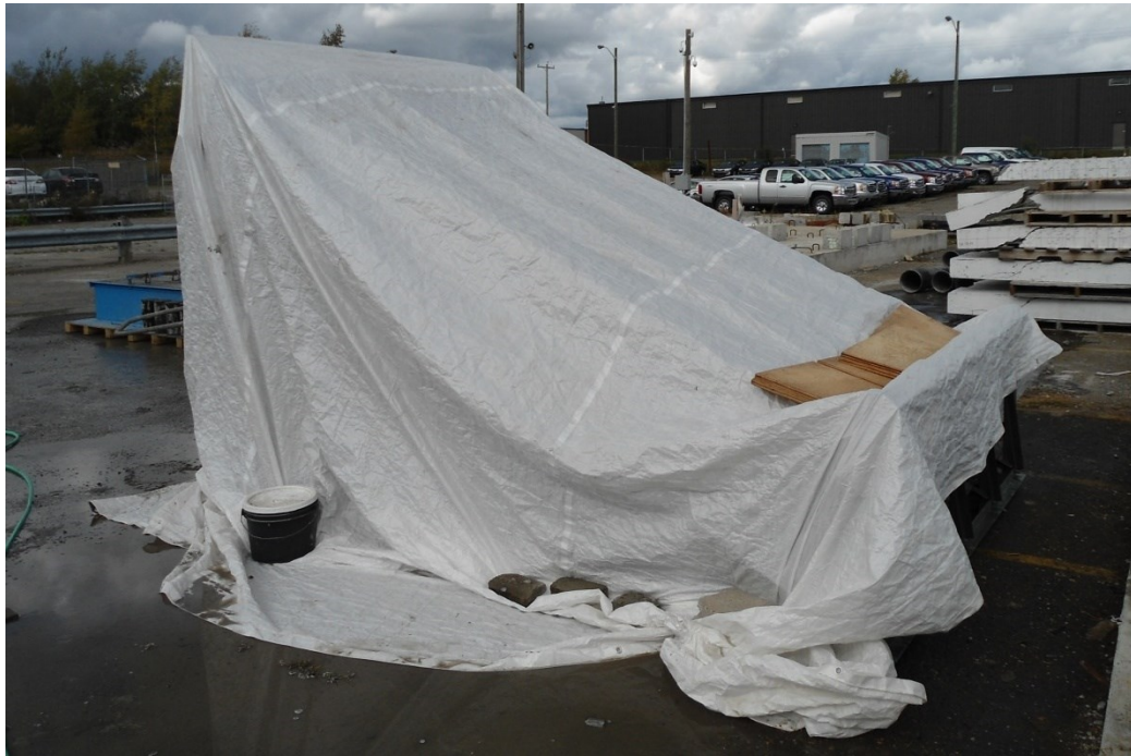
Figure 3.17 – Seven days moisture curing for CFFT beams
