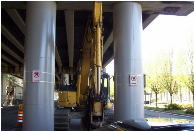
(a) CFFT columns in bridges
