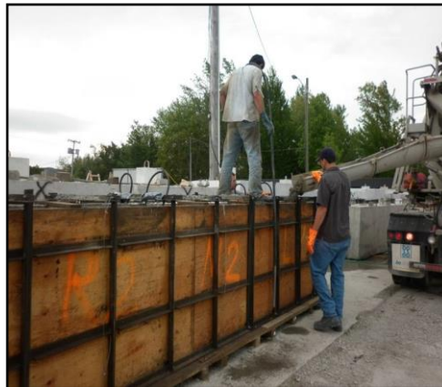
Figure 3.6 - Placement of concrete
