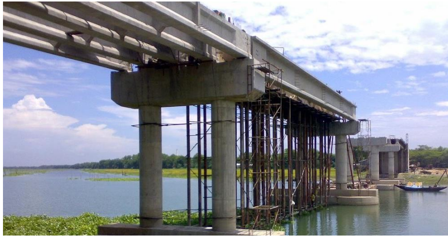
Figure 1.1 - Deep beam as transfer girder in bridges
