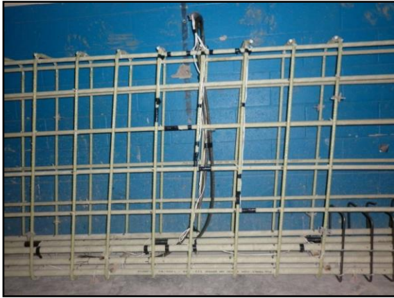
Figure 3.13 - FRP strain gauge for GVH-1.13
