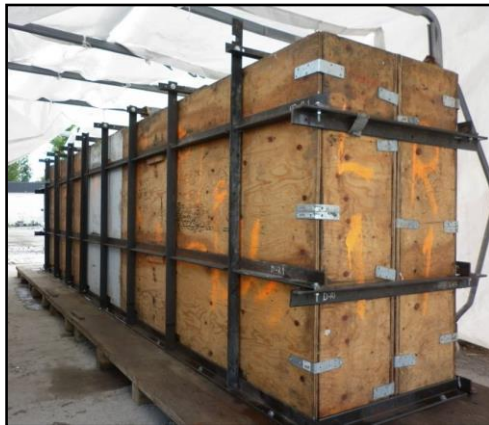
Figure 3.5 - Formwork in place prior to concrete placement
