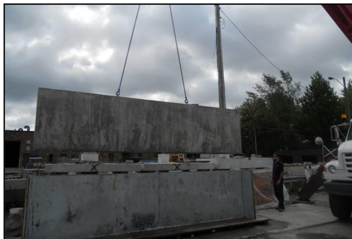
Figure 3.9 - De-molding of specimens using 25-ton crane truck
