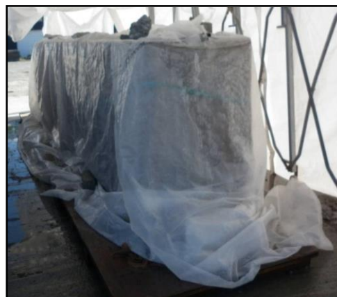
Figure 3.8 - Curing of concrete
