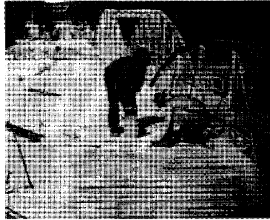
Fig. 2.1. Grouting of steel bars in bridge deck slab, Finland (Asplund 1949)
