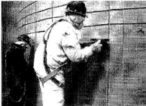
a) cutting the groove with a concrete saw. b) adding the adhesive material to the groove.
