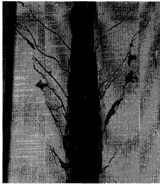
f) concrete tension failure with longitudinal and transverse cracks in epoxy (D-E-2.0-24)
