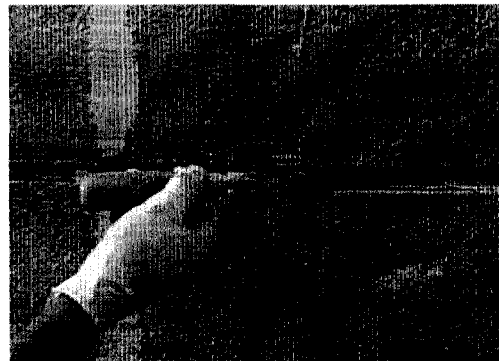
a) cutting the groove with a concrete saw. b) adding the adhesive material to the groove.
