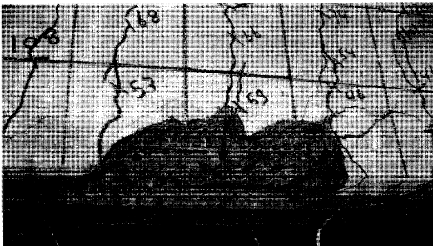
Fig. 5.11. Concrete cover split for B2
