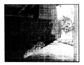
Figure 2.15: AAR-Induced Map-cracking in Components at St. Lambert Lock
