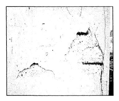
Figure 2.19: Spalling Exhibited in Component of Jacques-Cartier Bridge
