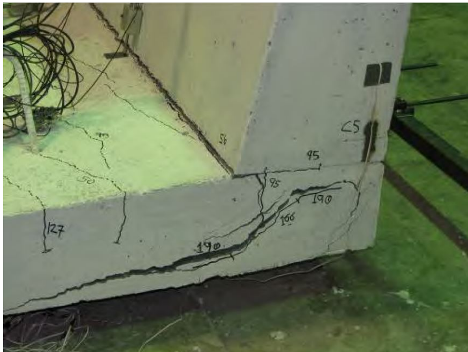
Figure 3.36 Mode de rupture du dispositif S-1650, [Ahmed et al. , 2010]
