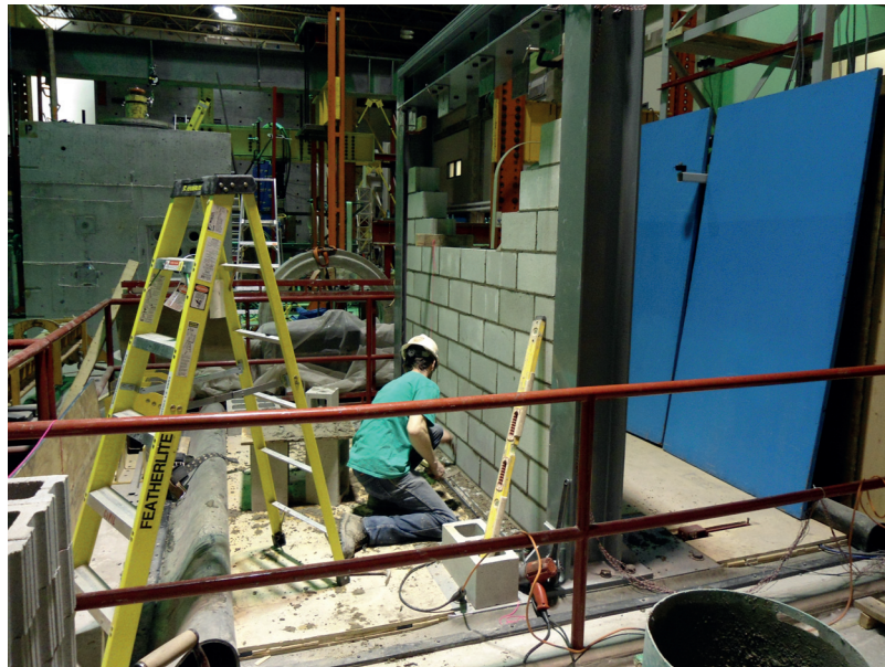
Figure A.8 Tirage de joints - Mur 2
