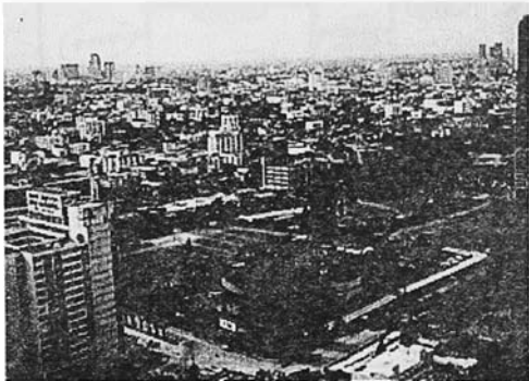
View from the south, Ramav9 Street: the back of the building and the service entrance (the left corner)/parking area at the front of the building (the right corner).
