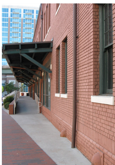
east portico from street level
