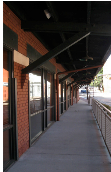
east portico from ramp
