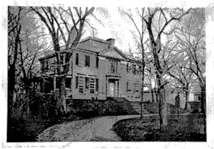
57. Taylor House , Roxbury, ca. 1790, Roxbury, Massachusetts. (Illustrated in William Rotch Ware, The Georgian Period: Being photographs and measured drawings of Colonial work with text . U.P.C. Book Company, 1923, plate 73.)
