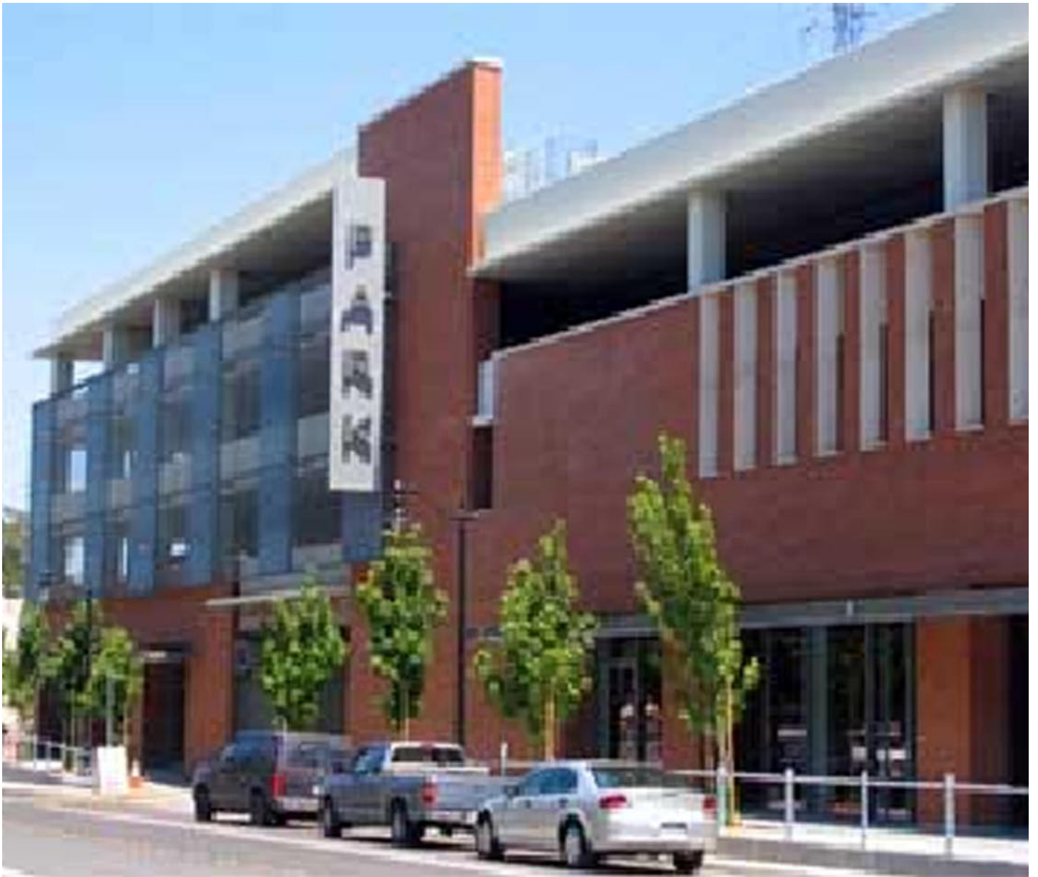
Petaluma, CA public parking garage
