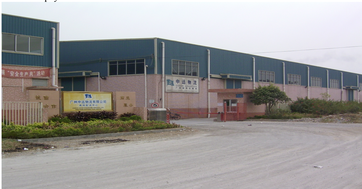
Procter & Gamble Zhong Yuan Wu Liu Company South District Distribution Center
