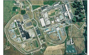
A bird's eye view of the Washington State Reformatory
