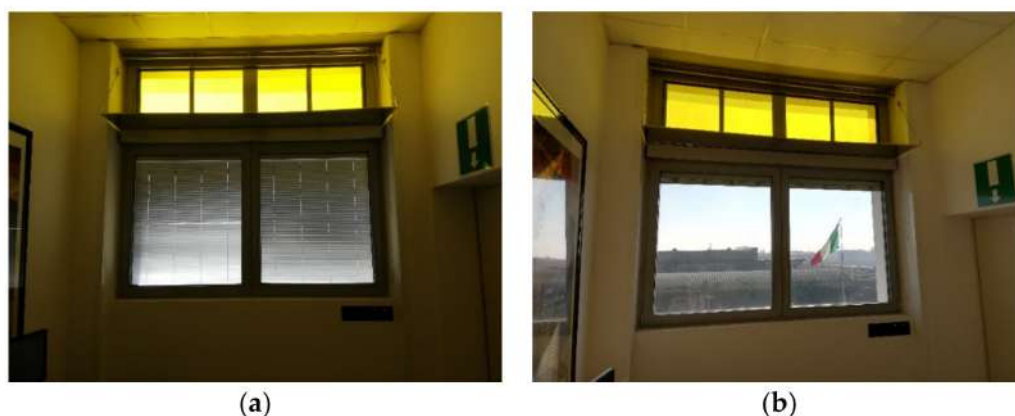
Figure 7. (a) Shading system in the configuration of the window completely closed. (b) Shading system in the configuration of the window completely opened.
