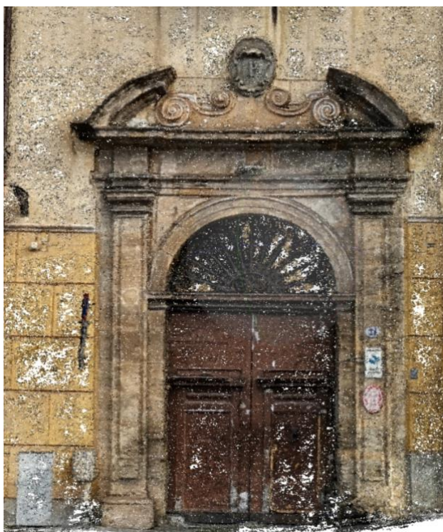
Figure 10: SfM reconstruction using low- resolution image of the portal of the façade of the ancient building. Dense Cloud
