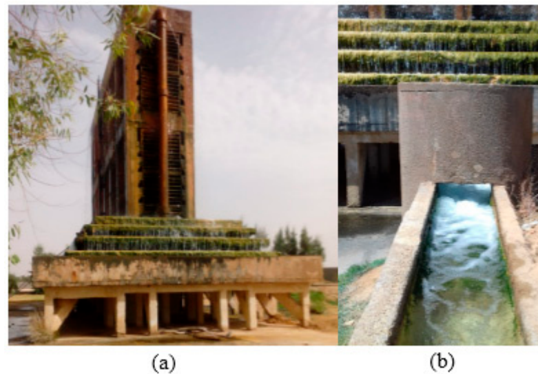
Figure 2. (a) Cooling system (b) irrigation canal.
