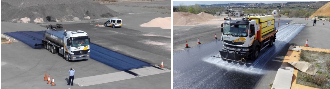
Figure 1. Application of tack coats in the experimental section, (a) with emulsion and (b) with emulsion and lime slurry.
