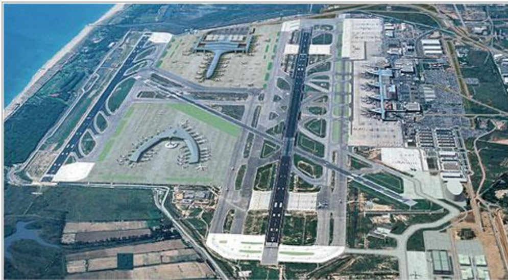
Figure 54: Potential map of the BCN airport with the satellite terminal (Source: GTD Systems)
