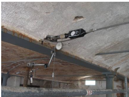
Experimental approach – Carrying out experiments on structural members
