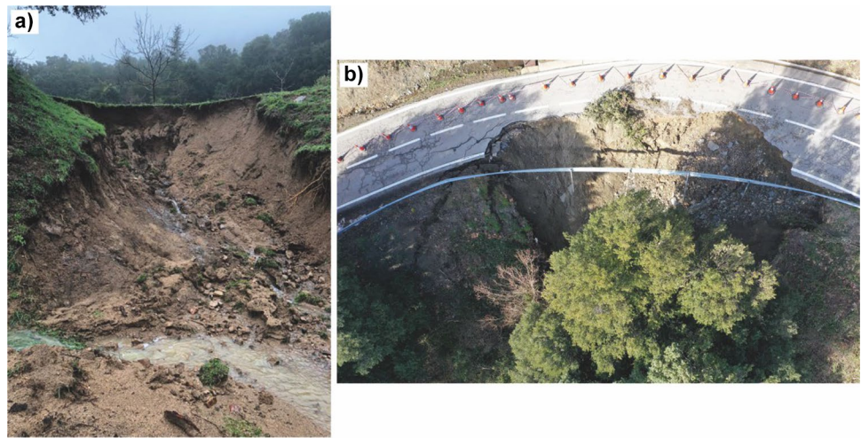
Fig. 7 Examples of landslides triggered by the Gloria storm in the Montseny area. a Rotational slide in a colluvium slope (photo courtesy of Clàudia Abancó). b Rotational slide that affected a road embankment and parts of natural slopes (photo courtesy of Roger Ruiz)
