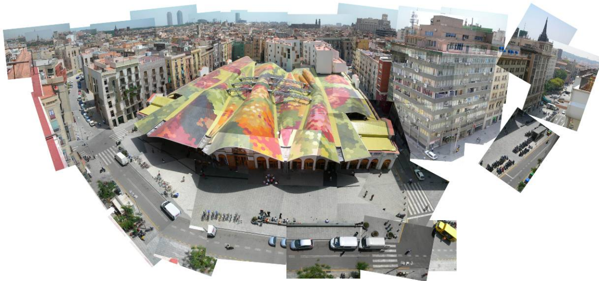
Figure 5: Top of the roof – Santa Caterina market, Enric Miralles and Benedetta Tagliabue, Barcelona, 2005 [Photo courtesy: EMBT architects].
