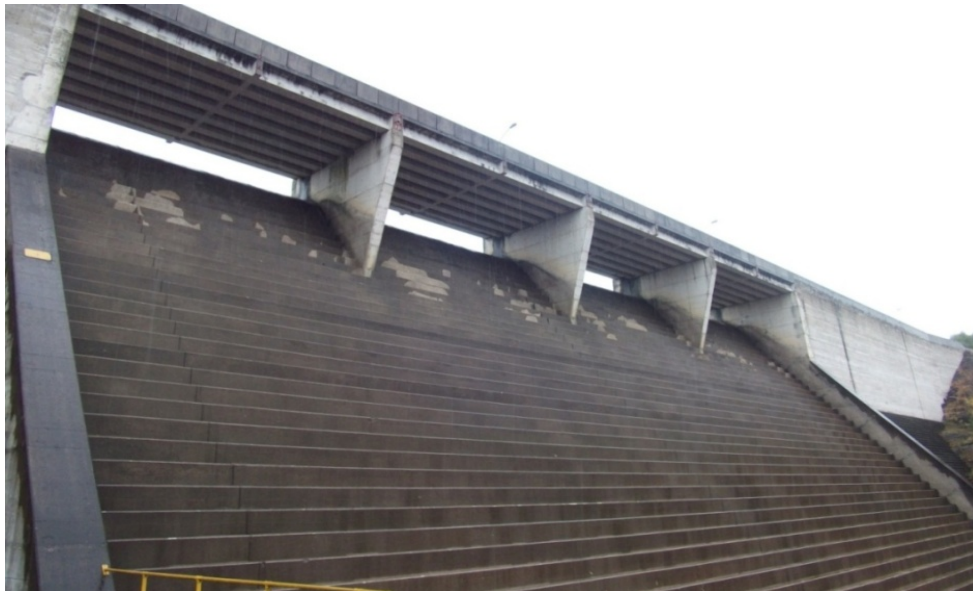
Figure 2. View of the structure of energy dissipation.
