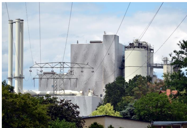
Figure 13: Cogeneration plant Cottbus, Picture: Trio3D [CC BY-SA 4.0 (https://creativecommons.org/licenses/by-sa/4.0)].
