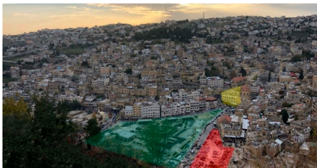
Figure 7. Oqbe Bin Nafe' project phase 1 highlighted in green, phase 2 highlighted in red and phase 3 highlighted in yellow [34].
