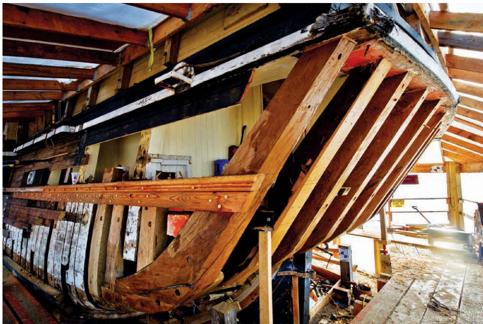
Structural work in progress on the Morgan's stern in November 2012
