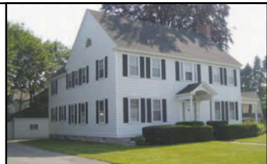
This 5 BR, 3 1/2 bath colonial offers formal in-town living a block from waterfront shopping & dining. Restored & upgraded throughout preserving wood floors & the charm & character of the era. New granite kitchen, heat, electrical, roof & more! Rockland $449,350
