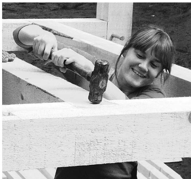
Marnie Briggs of Bath assembles a mortise-and-tenon joint.
