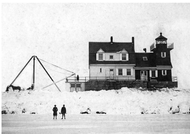
A nearly photo of the Rockland Breakwater Lighthouse
