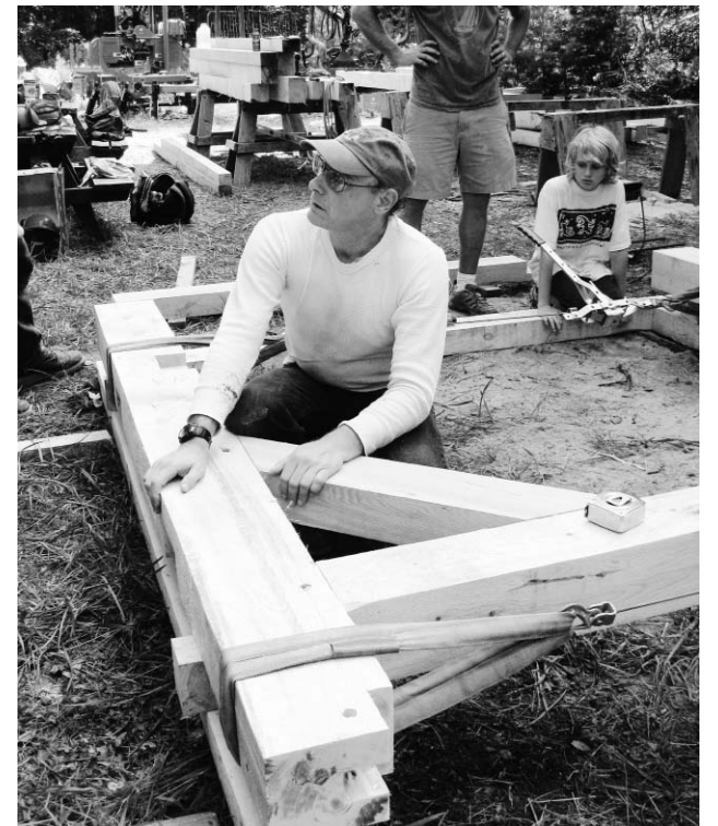
David Jenney inspects the timber-frame joint.
