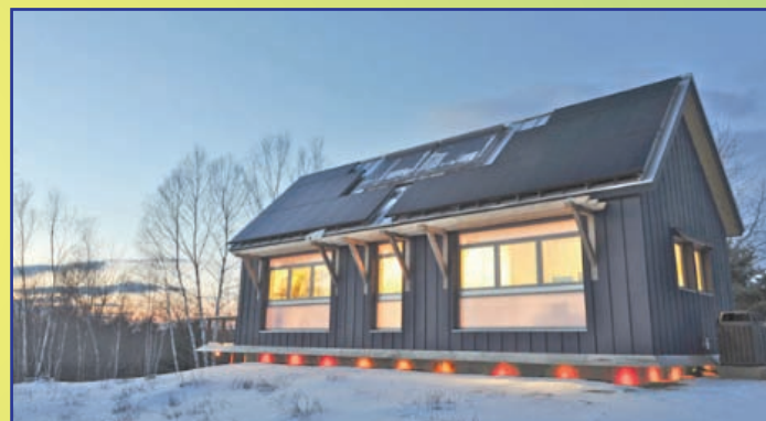
Exterior lighting glows green when energy flows back to the grid and red when receiving power back from the grid.
