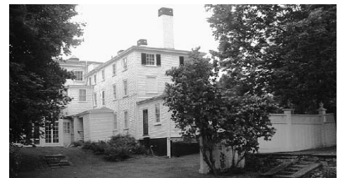
The Nickels-Sortwell House from the back garden PHOTO COURTESY HISTORIC NEW ENGLAND
