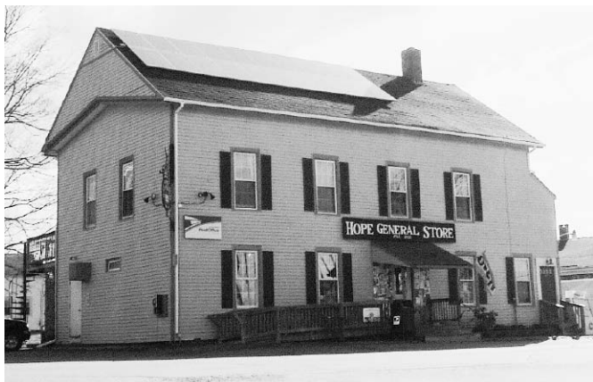
Hope General Store has a new 4.6-kilowatt grid-tied solar electric system.
