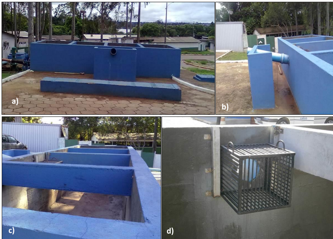
Figure 2: Detailed photographs of the Pilot Plant: a) front view of the equalization tank; b) entrance of the tank, access to the hoses of the trucks; c) view from inside the tank; d) box-shaped grid at the entrance to the tank.
