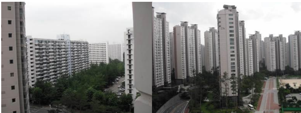
(a) Unreconstructed 5 th complex (b) Recently reconstructed 2 nd complex
