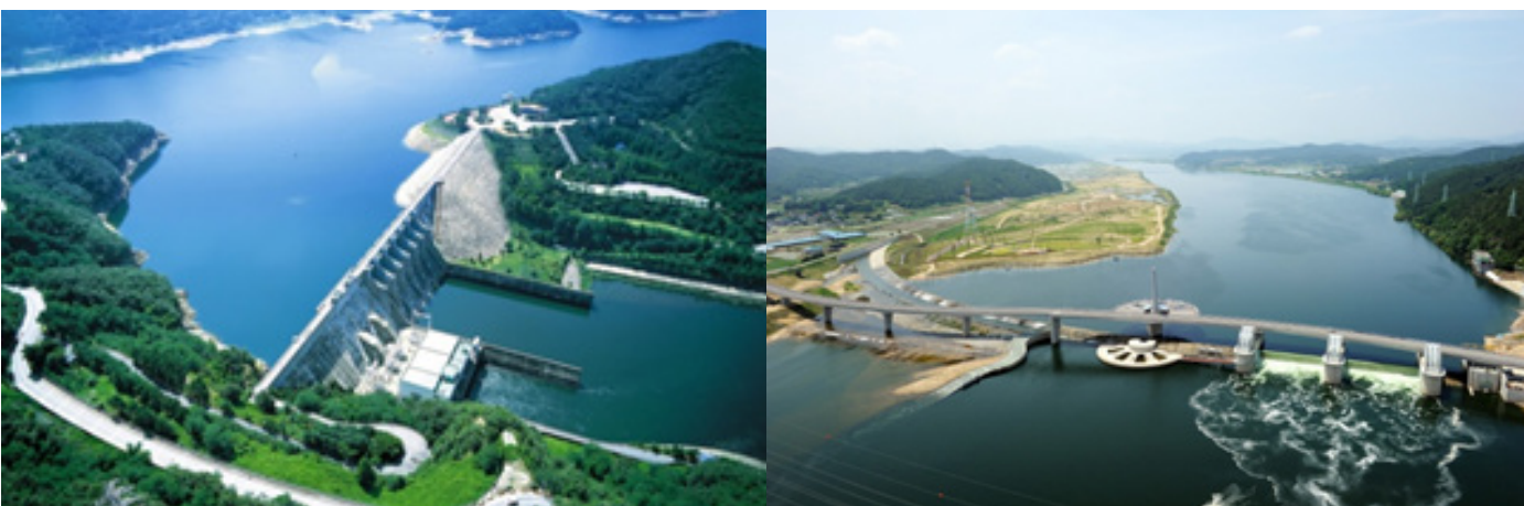
Figure 2. Dae-cheong dam reservoir (left) and Nak-dong river and its weir (right)
